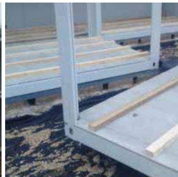
Module placement on 10kN blocks
