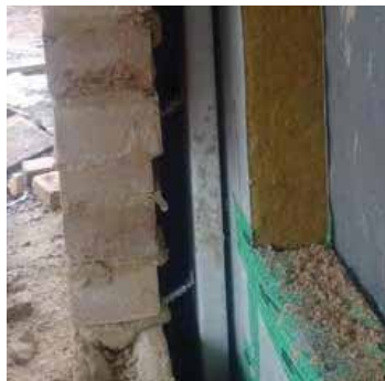
Brick tie connection
