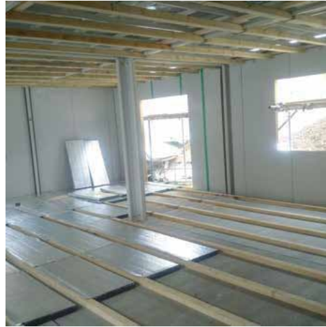
Insulation under floating floor
