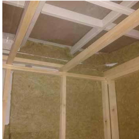
Showing first layer of insulation prior to the rolled insulation being fitted
